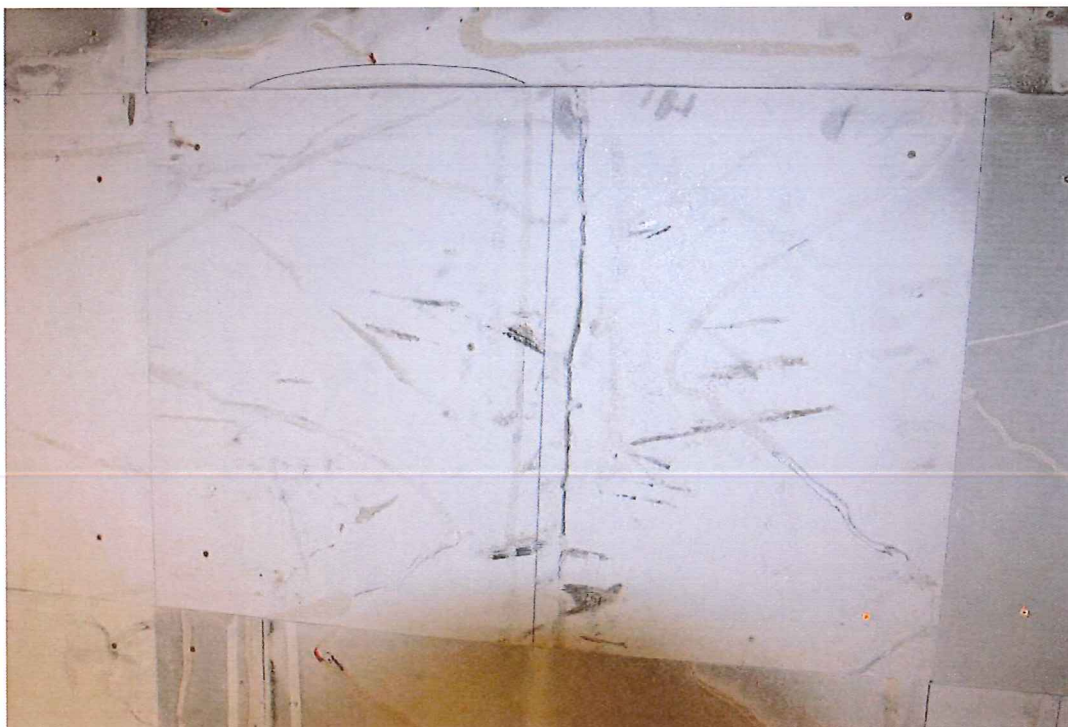
Figure 1. Calcium silicate board screwed to wall of fire test room
