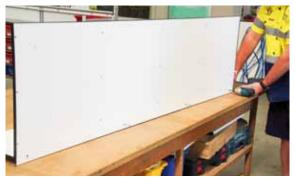
Fix top and bottom panels into side and back rebates. Top panels may have holes for coat hook.
